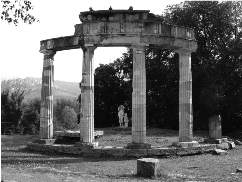
Figure 13.5. The second-century AD round structure of the nymphaeum in Hadrian's Villa at Tivoli. Photo courtesy A. Pollini.
